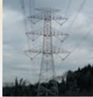
500kV系送電の実運用 こと Epoch-making New Technology, The First 500kV Transmission Line Ever Constructed in Japan モノ
