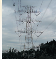
ごうりゅうけんぱんぱん 500kV系送電の実運用 Epoch-making New Technology: The First 500kV Transmission Line Ever Constructed in Japan
