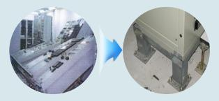
Application of seismic reinforcement technologies (765kV substation facilities, etc.)
